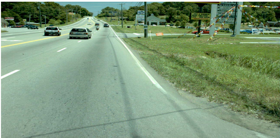
End of project. US 441 (State Route 71) at Macon Lane looking back toward the beginning of project. Note drainage ditch to the right for that may need to be relocated to maintain drainage at LM 29.94.
